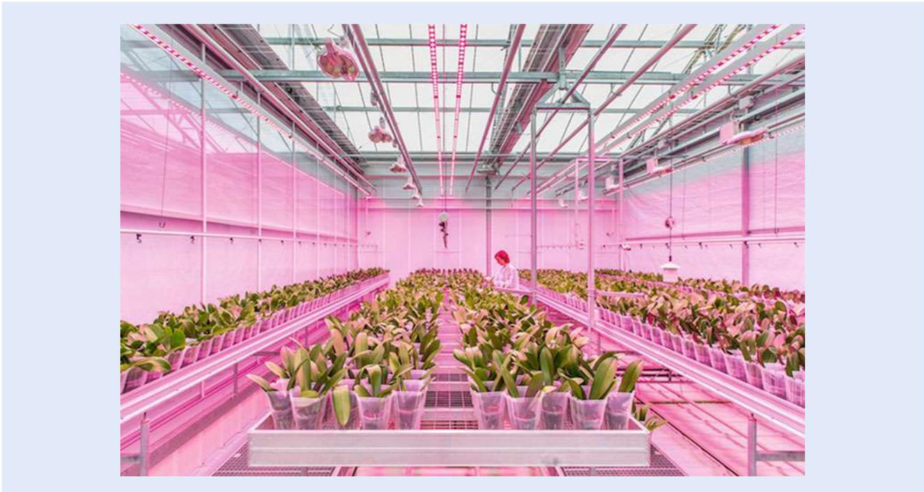
■ Fig. 5.23 Philips LED lighting for fast-track growth in horticulture. Image from Philips, with permission
