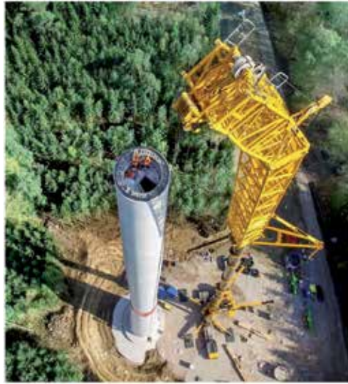
Figure 9. Installation of the internal steel tower by means of a crane (Credit: Max Bögl).
