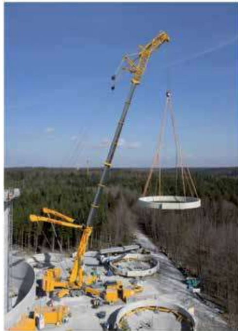
Figure 7. Putting together concrete rings at the construction site by means of the Liebherr 630 EC-H70 self-erecting slewing crane (Credit: Liebherr Plant Ehingen GmbH).
