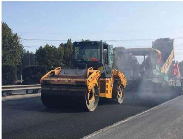
**Figure 5.** Mechanical equipment used for asphalt paving and compaction: pitch paver and road roller.
