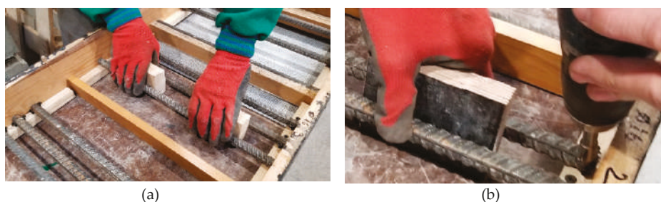
Figure 7. Stabilization of reinforcement in formwork: (a) distance resulting from wooden spacers, (b) rebar fastening to wooden washers with screws.
