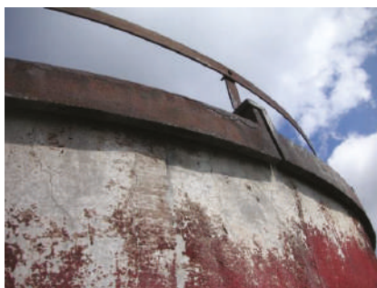
Figure 3. Condensation dripping down from a chimney upper ring.
