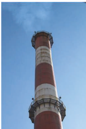
Figure 1. Deposition of condensation on outer surface chimney wall along construction joints.
