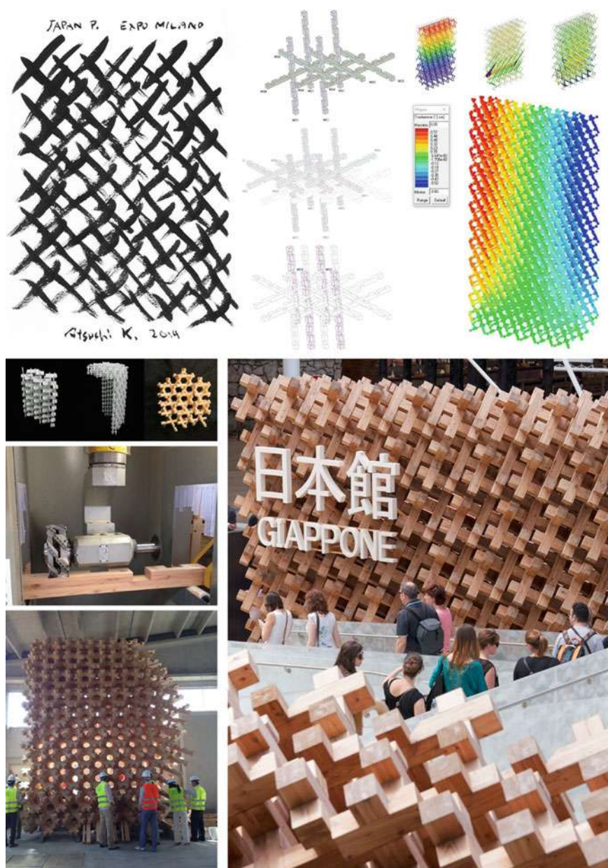
Fig. 1 Japan Pavilion wooden façade, conceived and realized for EXPO Milano 2015, thanks to an intense and iterative process between computational and parametric design, FEM-based structural analysis and digital fabrication with CNC machines, which allow both real scale mock-ups and final fast and precise assembling on site ( drawings and photo courtesy Atsushi Kitagawara Architects and Galloppini Legnami )
