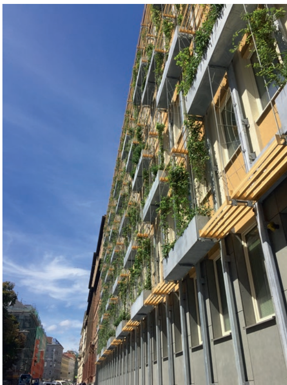
Fig. 10.9 Green wall takes on the function of external shading. Retrofitted building from the 60ies. MA 31 Vienna (Source: Vera Enzi)
