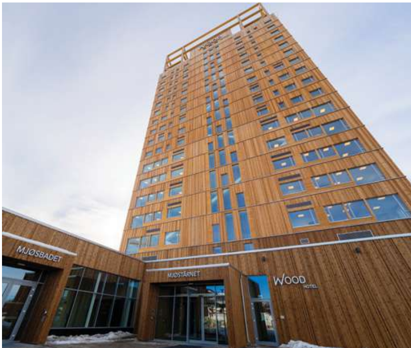
Figure 4 The 85-meter-high Mjøstårnet in Norway. The building’s structure is composed of both glued laminated timber and cross-laminated timber
