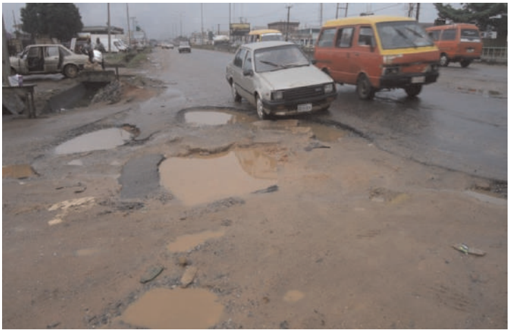
Figure 4. Showing how water aids road failure.
