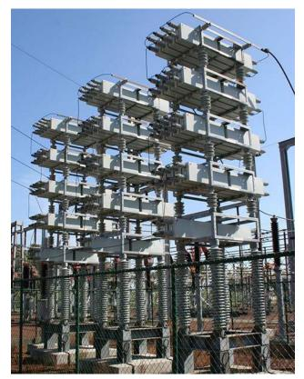
Figure 15.14 Power capacitors are used to balance the impedance of the effective inductance in transmission lines.
