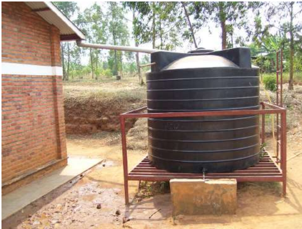
Figure 4.14: Rainwater harvesting storage tank example.
