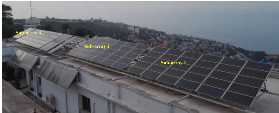
Fig. 4. Grid connected photovoltaic generator on roof.
