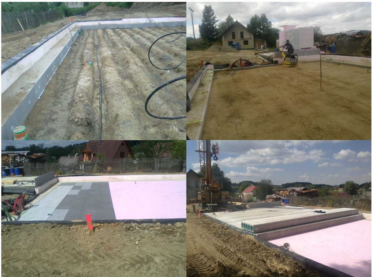
Fig. 2. Realization of low-cost ground storage within foundations.
