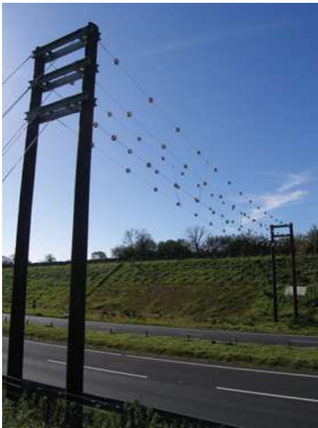
Figure 4.3 Two bat gantry designs: (a) wire mesh design on the A11, Norfolk, UK; (b) wire and ball design on the A590, Cumbria, UK. Boxplots show the results of surveys carried out to test the effectiveness of the gantries in guiding bats safely over the road. Data were recorded for the total number of bats crossing per survey, the numbers crossing at unsafe heights (below 5 m, traffic height) and the numbers using the gantry according to two definitions of ‘use’ (flying within either 2 m or 5 m of the wires above traffic height). The bat gantry story neatly demonstrates the need to test conservation interventions before rolling them out on a wide scale. From Berthinussen and Altringham (2012b, 2015). (A black and white version of this figure will appear in some formats.)
