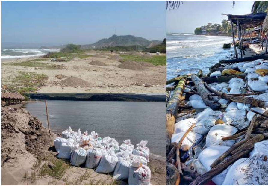
FIG 7.8 Throughout South America, sandbagging is common both for means of small operators handling illegal (or legal) mining and transport ( left photo ), and for convenient construction units for building low-cost groins and seawalls ( right photo ) that are generally ineffective. In the background of the photo on the left, one can see a common small-scale mining operation in Colombia, with multiple piles of sand dug from pits in the back beach, low dunes, and overwash fans. Photos by Nelson Rangel-Buitrago.
