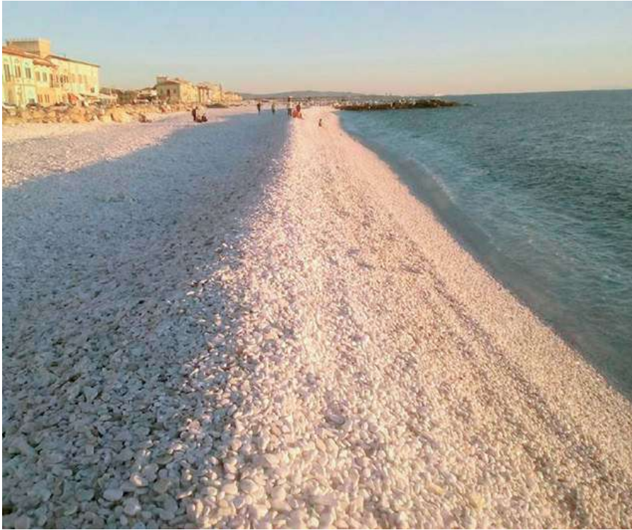
FIG 2.4 The pebble beach near Pisa, Italy, is a unique one that uses unusual materials for frequent nourishment. A nearby marble quarry furnishes a supply of scrap marble chips. A gravel beach may not be as comfortable as a sand beach, but it will do just fine because the chips are furnished at cost, and the beach is a good temporary buffer against sea level rise. Photo © Andrew Cooper.
