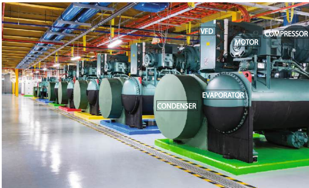
Figure 4.11: Water-cooled centrifugal chiller.
