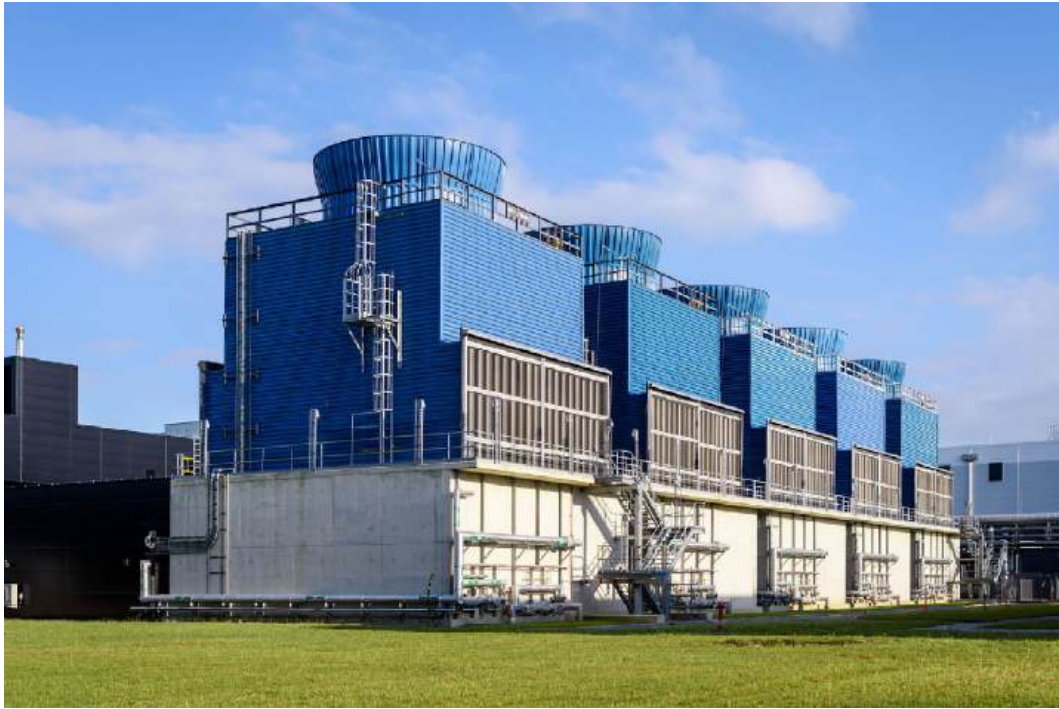
Figure 4.12: Data center cooling towers.
