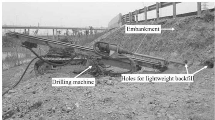
Figure 3. Drilling holes on north sides of the embankment. Reprinted with permission from Ref. [18]. Copyright 2021 IEEE Proceedings.
