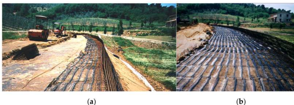
Figure 17. Geogrid reinforcement of a dyke with steepened slope in Tuscany (Italy) (a) edge of the slope and (b) flat area.
