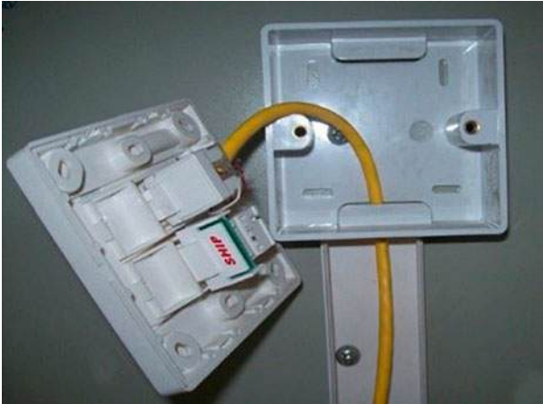
Fig. 2.41 Information module fixed on the back of the panel
