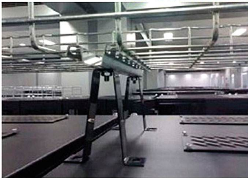
Fig. 2.64 Installation of supporting bridge for rack
