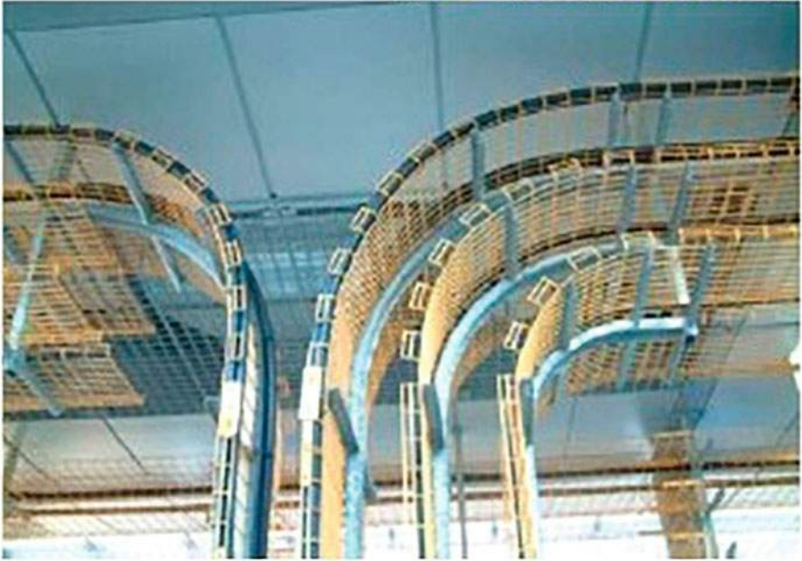
Fig. 2.63 Layered installation of bridges
