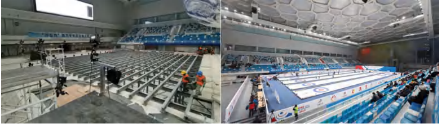
Fig. 1. Demonstrator DfD-based project of the Olympic curling hall in the Chinese National Aquatics Center (“Water-Cube”). The steel structure should be assembled and disassembled every year to accommodate the scenario changing requirement of the building
