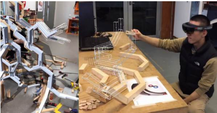
Fig. 6. The aggregation was assembled in chunks, and then together using a series of holographic guides
