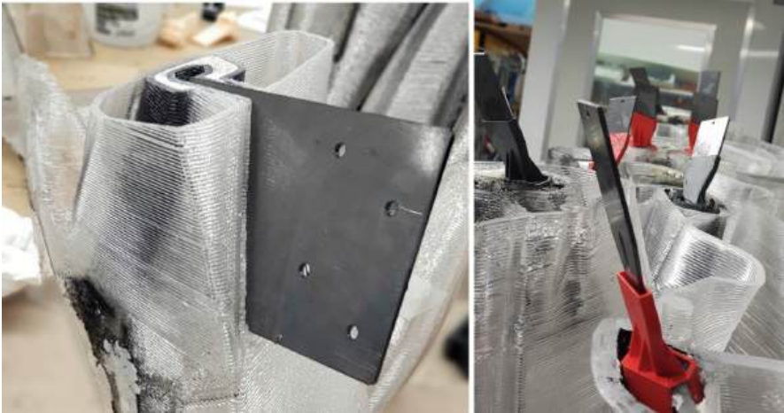
Fig. 11. Steel plate wall connection (left), implanted steel connections (right)
