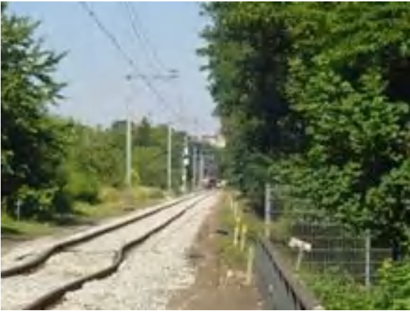
Figure 3.12.2 Buckling of tracks (Wikipedia)
