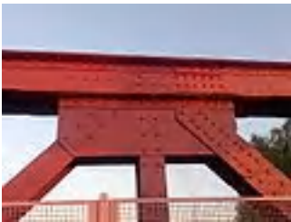
Figure 6.2 Member connections (from Wikimedia Commons)
