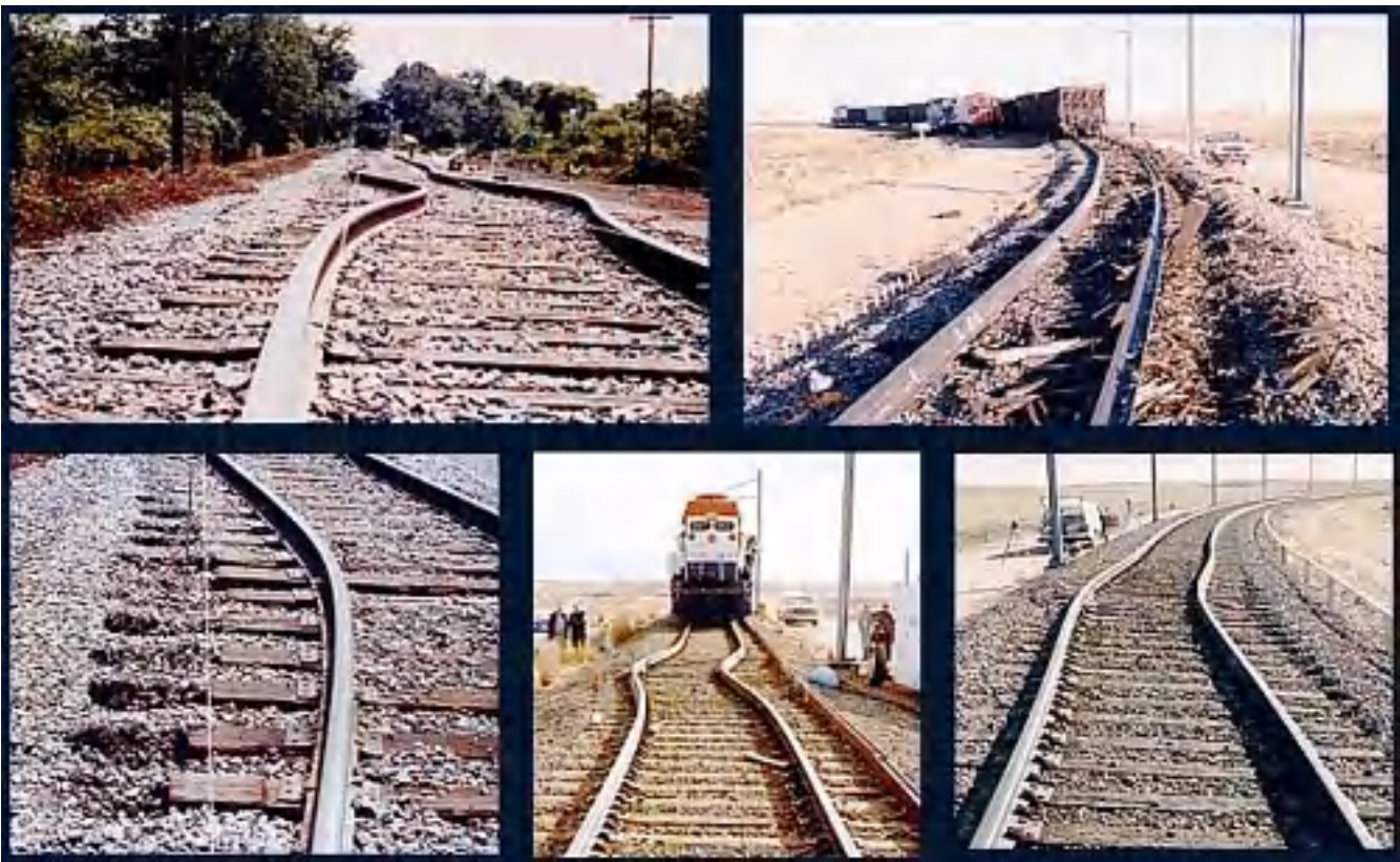
Figure 3.3.1 Buckling of railroad tracks - thermal strain (Courtesy of US Department of transportation - Volpe Center)
