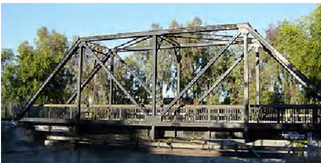
Example 6.2.1 A simple bridge truss -and simplified.
