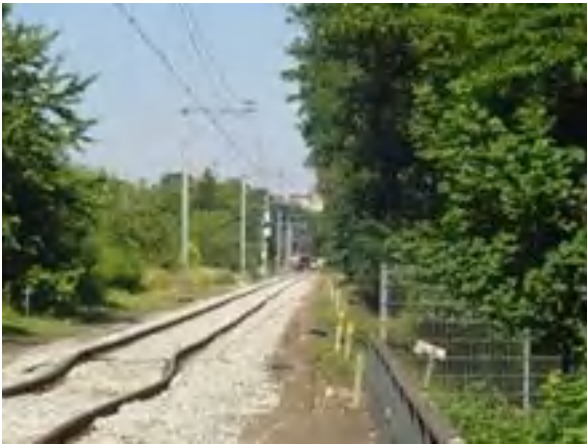
Figure 9.2 Buckling of tracks (Wikipedia)
