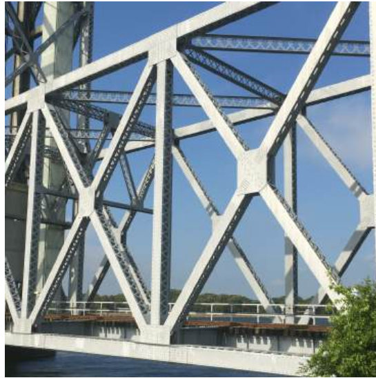
Figure 6.3.1 Truss with riveted gusset plates.
