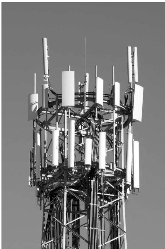
Figure 2.25: The antenna tower of a modern cellular site, supporting several UHF and SHF-band cellular systems.
