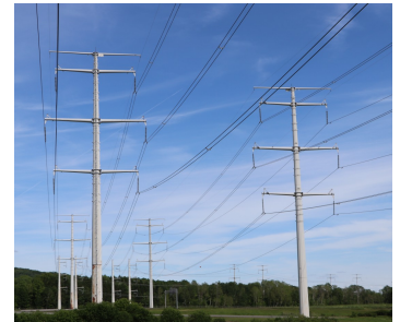
Figure 1.1 345,000 volt transmission lines.
