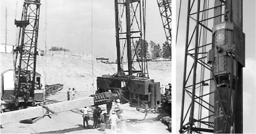
**Fig. 5.3** (Left) Job site during preparation to drive a pile using resonant excitation provided by two engines from a Sherman tank. The engines provided counterrotation of eccentric masses (see Fig. 5.4) that drove the pile at its longitudinal standing wave resonance frequency. (Right) A 140 kW (200 HP) resonant driver, mounted on a 60 cm diameter steel pile, that uses a high-speed hydraulic valve to drive the pile at resonance. (Photographs courtesy of Matthew Janes)
