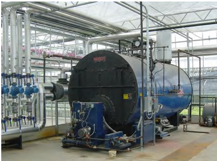
Figure 8. Hot water heating system including a boiler, mixing valves, pumps, and distribution plumbing (Photo by A. J. Both).
