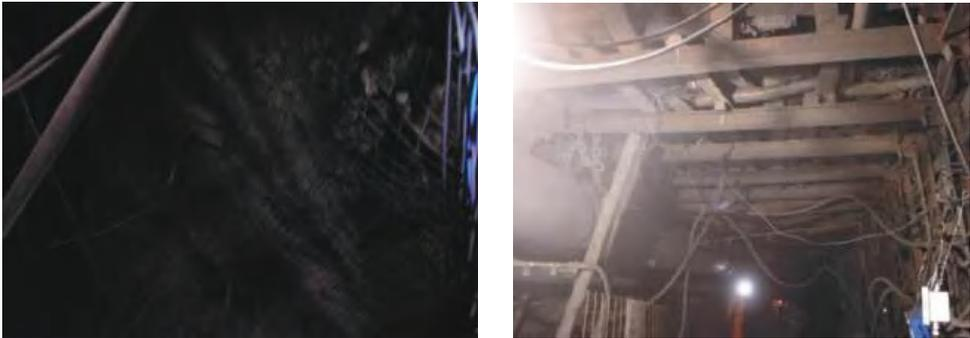
Figure 4. Deformation of surrounding rock during roadway excavation.
