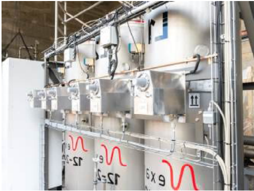
Figure 9.1.4: 10 kV, 40 MVA resistive type superconducting fault current limiter [Schmidt2015]
