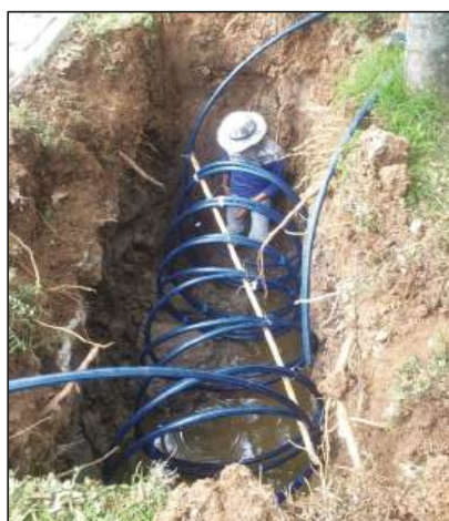
Figure 6. Installation of a helically configured heat exchanger (Group 4).
