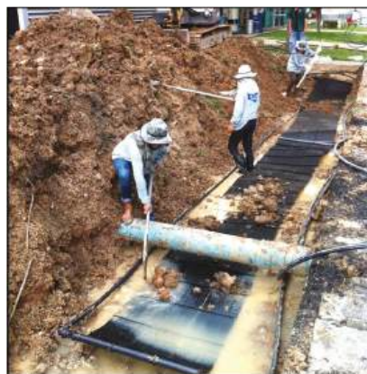
Figure 4. Carpet-type heat exchanger installation.
