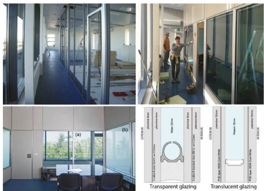
Figure 2. Top: View from the access corridor during the construction process. Bottom: Glass configuration of the office space. (a) Transparent Water-Flow Glazing (corridor), (b) translucent Water-Flow Glazing (interior partitions).
