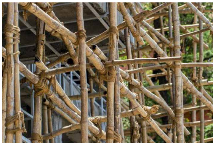
Figure 1. Bamboo culms used for scaffolding.
