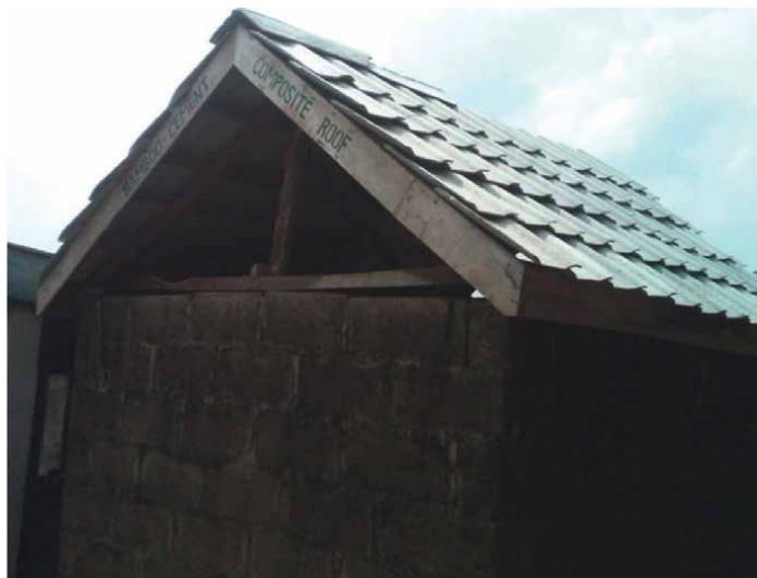
Figure 12. Bamboo-cement roofing tiles installation.
