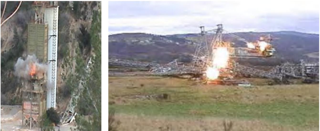
**Figure 5.** Demolition of metallic structures with shaped charges ((left) metallic silo; (right) large mining stacker).
