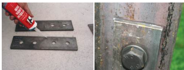
Figure 8. Application of silicone sealant ((left) application of sealant to the splices; (right) sealant smoothed around the perimeter of the splice).
