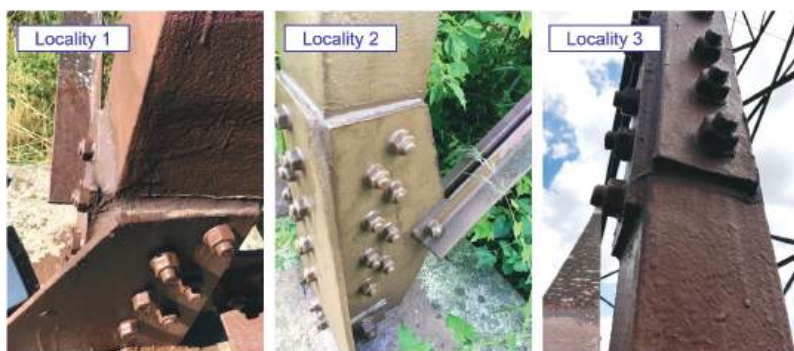
Figure 18. Functional crevice protection with sealant (selected examples).
