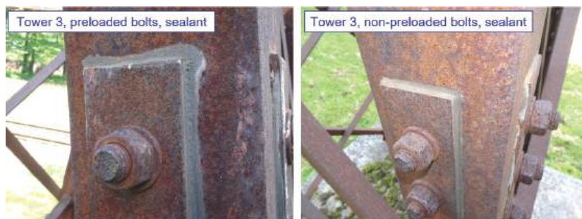
Figure 23. Tower 3: Selected examples of joints (functional sealant along the edge of the splice).
