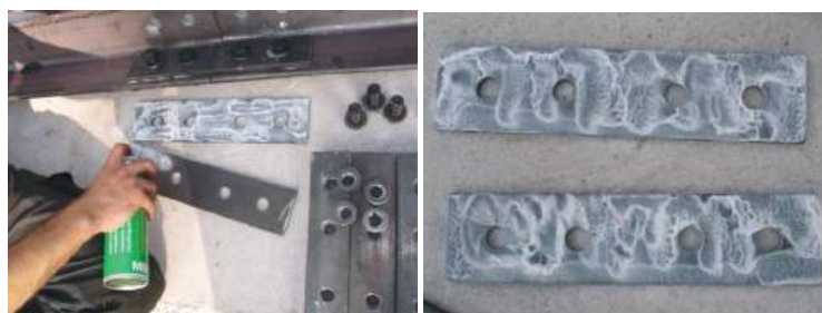
Figure 9. Application of Teflon Vaseline to the splices.
