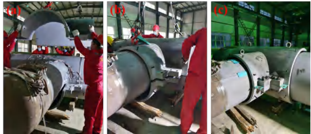
Figure 8. Installation process of special-shaped steel sleeves: (a) positioning, (b) gap adjustment, and (c) bolt fastening.
