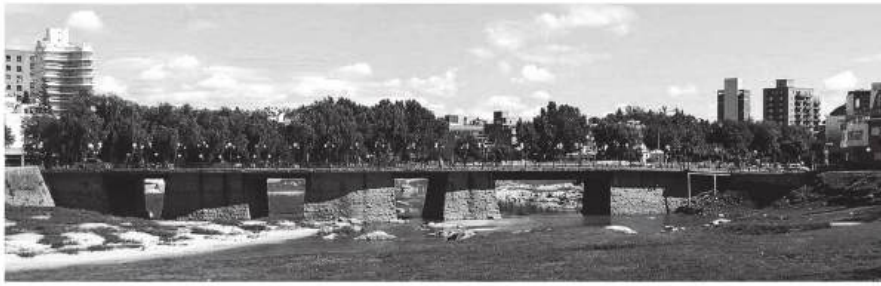
Figure 2. The existing 1889 bridge, its supporting piles account for 45% of the drainage section. (Credit: Reproduced with permission from the author, Eng. Gerónimo Cáffaro).
