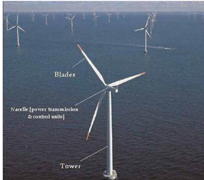
Figure 1. Horizontal-axis wind turbine system components.
