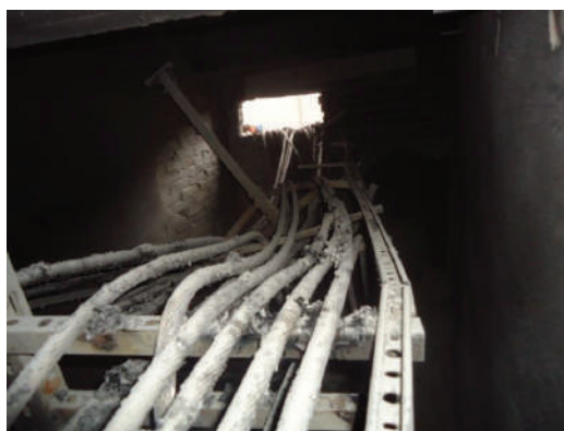
Figure 1. A destroyed cable supply system [16].
